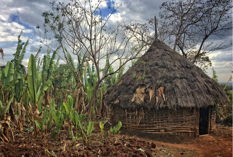
Figure 8: A local home with thatched roof
